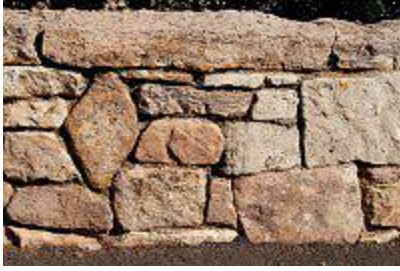
A portion of the stone wall.
